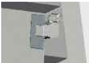
Sockelleiste/ baseboard ducts
